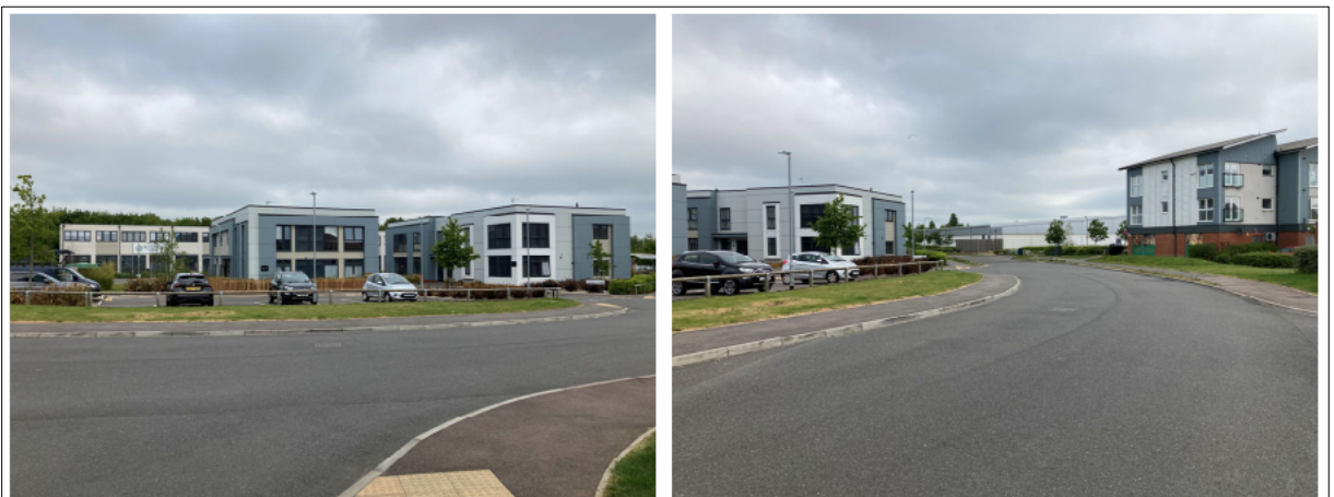
View looking to site from Hurricane Way
